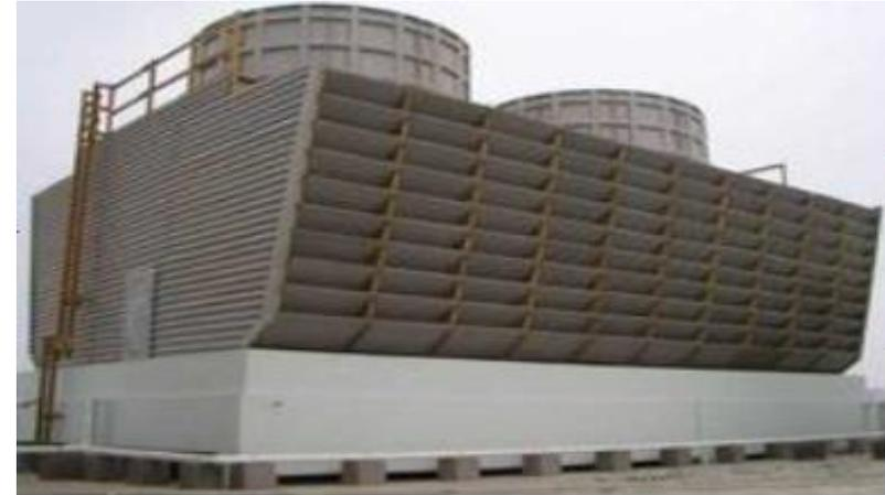
Water cooling tower for the blast furnace
